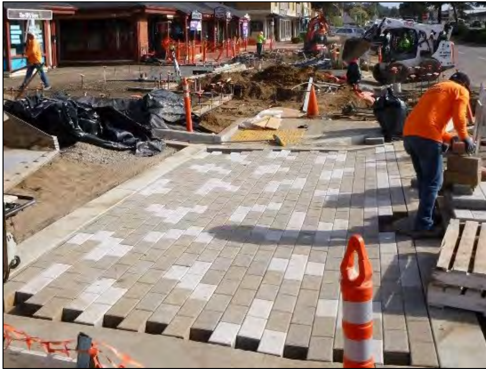
The installation of pavers at a crosswalk.
